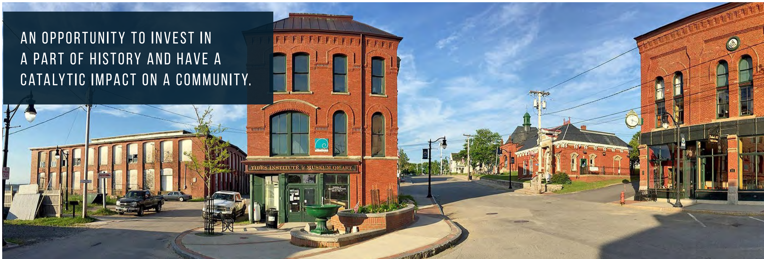
From left: American Can Co. (to be renovated), Tides Institute and Museum of Art (former Eastport Savings Bank), Peavey Memorial Library (a Carnegie Library), Business Rental (former Frontier National Bank), Masonic Block, presently under renovation.
